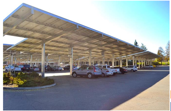
Example of solar carport
