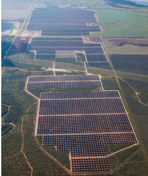
Alamo 7 Solar Farm 106.4 MW – Haskell, Texas
